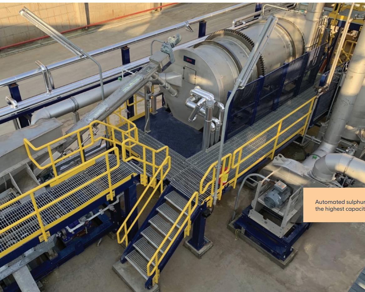
Automated sulphur granulation process with the highest capacity granulation unit available.
